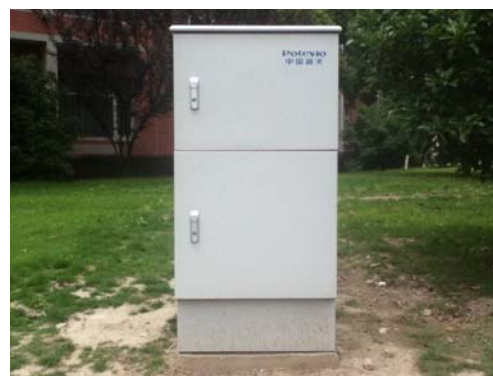
Figure 2 Charging pile integrated cabinet Electric vehicle data communications network platform frame shown in Figure 1. Pure electric cars and charging network access points will pile charging piles arranged in the vicinity, which is placed in the charging piles integrated cabinet (Figure 2) in. Integrated charging piles around the cabinet will be available through the vehicle charging piles internal wireless routers get connected to the wireless network, the router will also share their Internet connection to the vehicle users, and charge pile. Here, the router to get Internet connection, there are three main ways, one through a wired network (fiber-optic network, ordinary broadband networks, dedicated networks, etc.) to obtain Internet network connection, the second is to get Internet via 3G cellular networks network connection, three by 4G cellular network of Internet network connection. Pure electric car charging pile and can be obtained through these networks link the ability to connect with a remote server, allowing the recorded data itself is sent to the remote server database. Based on these data the remote server, you can think that pure electric car manufacturers to provide various customized data services.
